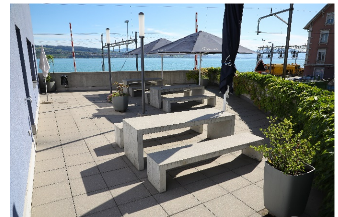
Restaurant Prager Terrasse
